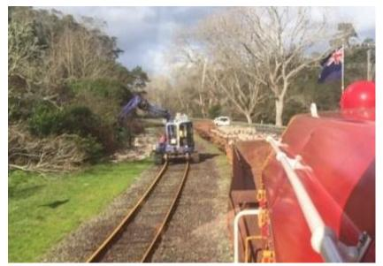
Recently Dean McQuoid, a member, through his contacts at KiwiRail, asked what KiwiRail was doing with the concrete sleepers that they were progressively replacing throughout their rail network. The sleepers were being replaced as they had reached 'their use by date' due to the speed and weight of trains running over them. For Goldfields Railway, the
